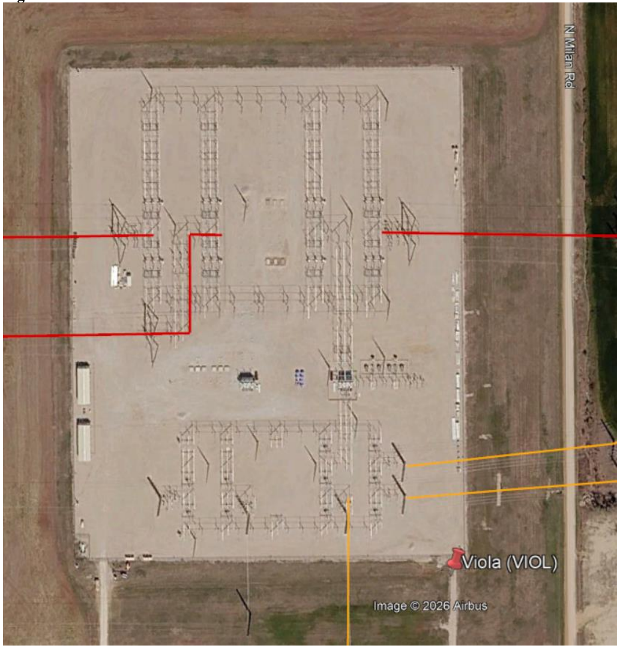
Figure 1 – Viola 138/345kV Substation
